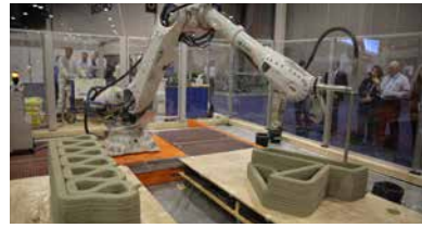
The impact and opportunities of automation in construction
