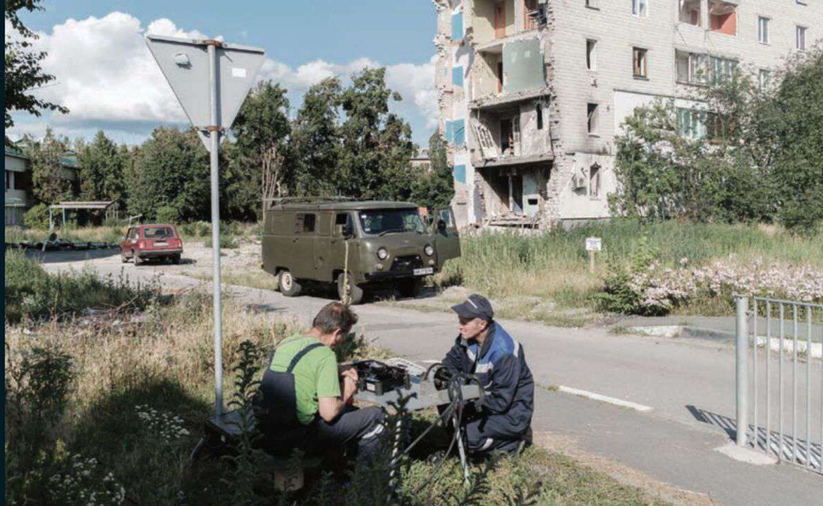
Ukrtelecom engineers in a battle-damaged part of Borodyanka
