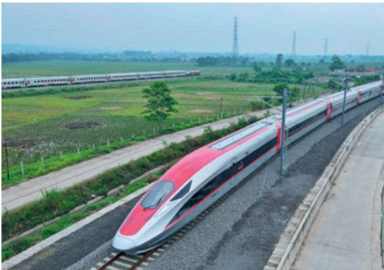
Electric multiple units conduct hot testing on the Jakarta-Bandung High-Speed Railway trial section in Bandung, Indonesia, on November 9
